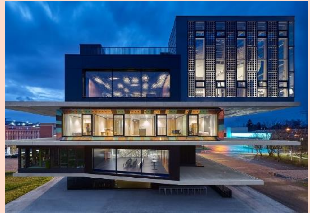
The Urban Mining and Recycling (UMAR) Experimental Unit is an experimental building mostly constructed with fully reusable, recyclable and compostable building materials.
