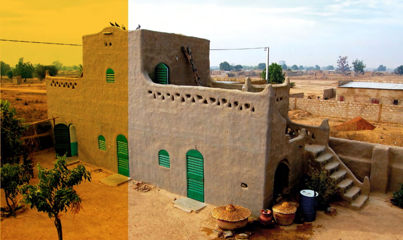
Examples of construction with a second storey.
