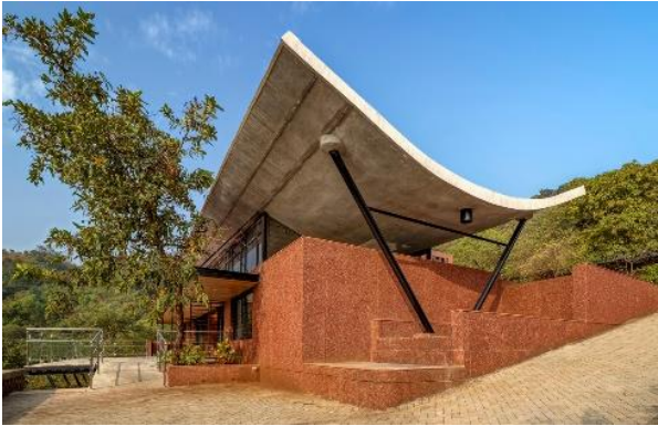
Figure 8: The cove house uses inverted roof to harvest the rainwater which is channeled and stored in multiple water bodies. (Architects: Red Brick Studio)
