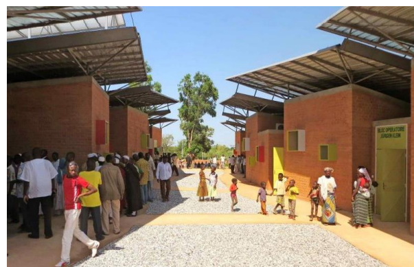
Figure 3: Léo Surgical Clinic and Health Centre uses passive cooling techniques such as compressed earth bricks and large overhanging roofs (Architects: Kéré Architecture)
